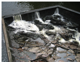
Main Street Dam
